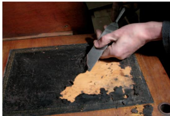
*Preparation* Dampen the old leather then remove it with a wide-bladed chisel (above). If you need to do any chamfering to the panel, first score the edge (right)
