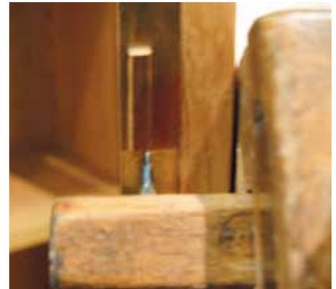
▲ Pic.39 ...to give the length and breadth of the lock bolt slot...
