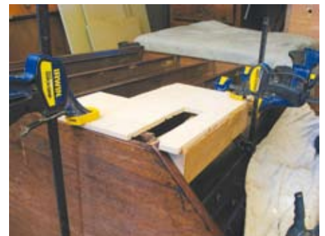
4 Preparation for cutting recess to repair broken hinge area
