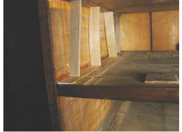
14 Fillet glued in place on dust boards using sprung lathes
