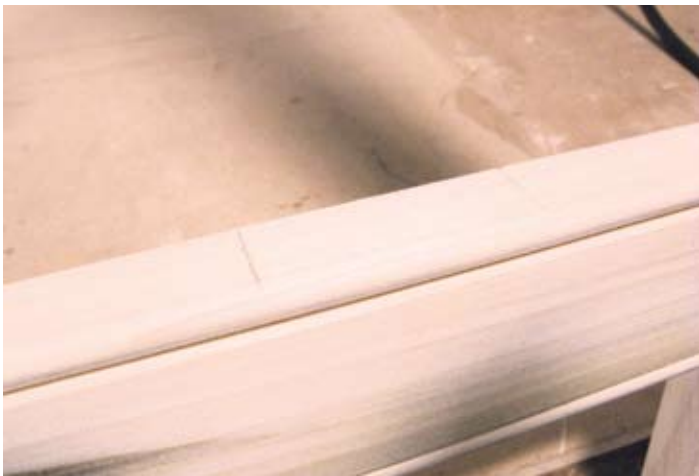
▲ Pic.13 Lightly square the marks across the frame using a pencil...
