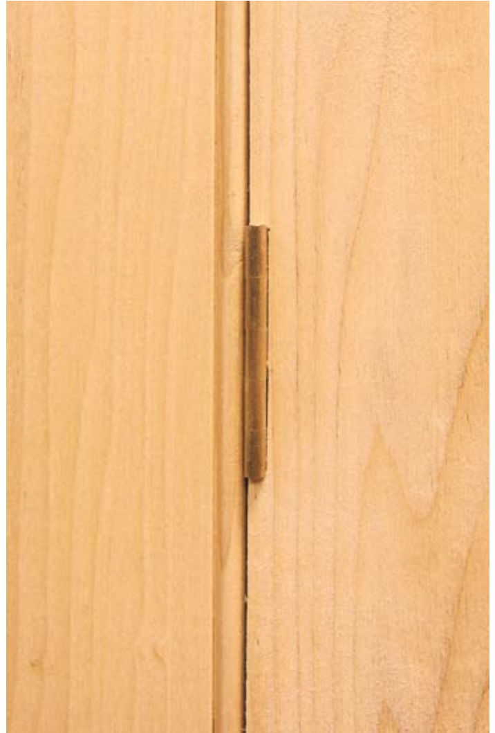
▲ Pic.19 The hinge could have been recessed into the frame bead, but here the vertical lines are uninterrupted
